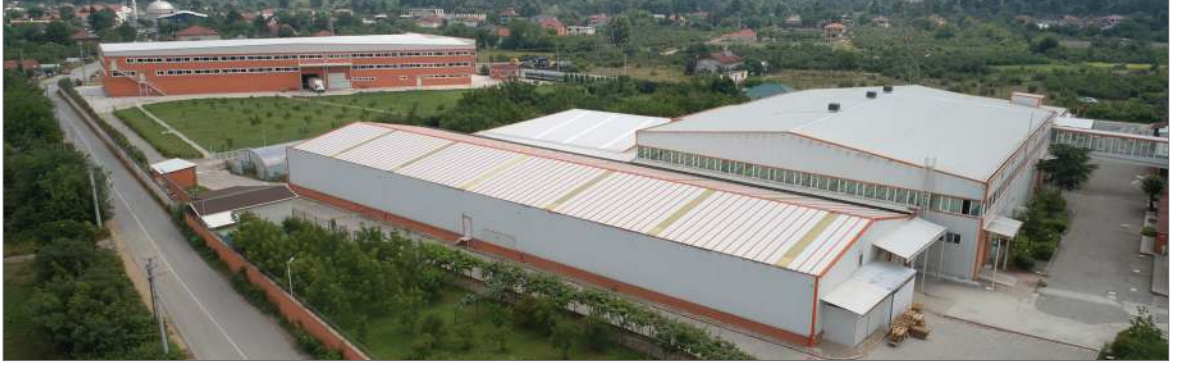
Ana Fabrika / Main Factory
